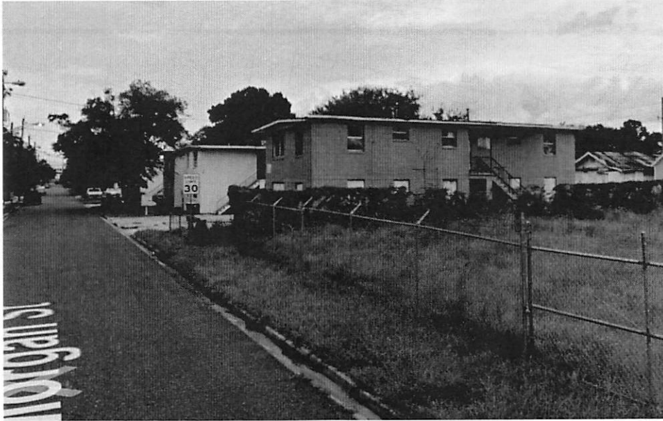
Adjacent multi-family to the east, along Morgan Street
